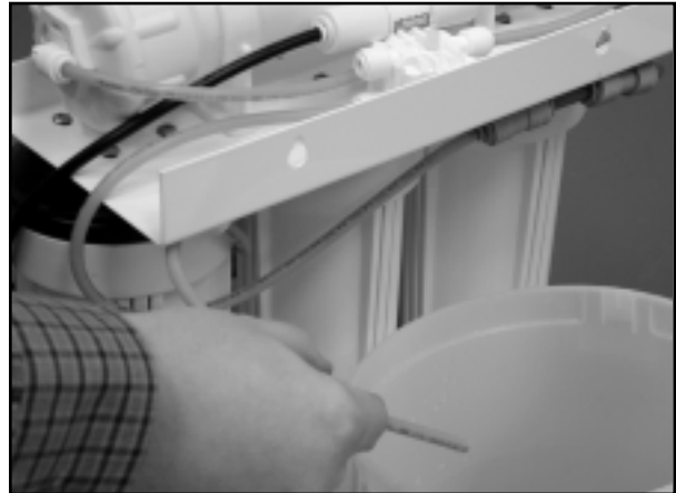
Figure 11 - Direct flushed water and carbon fines into container
